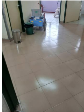
Tiled floor - easier to maintain in a hot and humid climate
